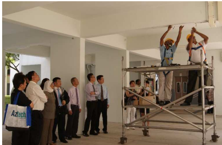
Installation of LED lights at one of the housing blocks.
