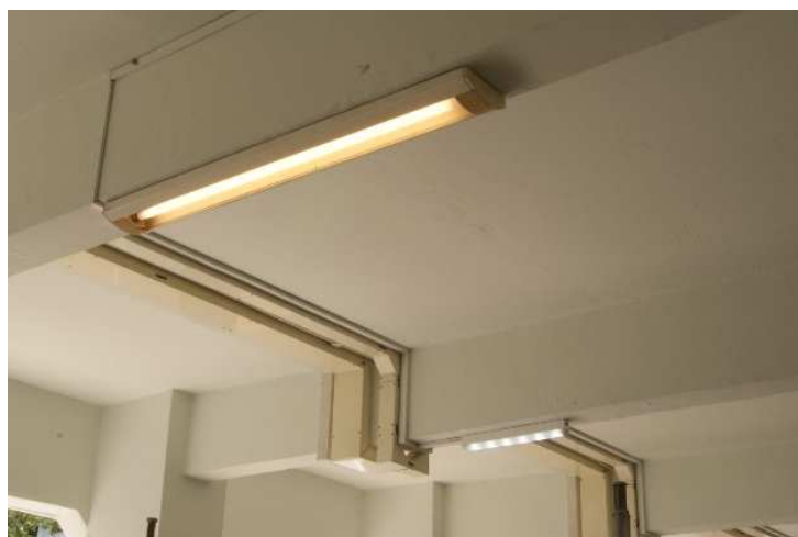
Fluorescent lights (left) versus LED lights (right).
